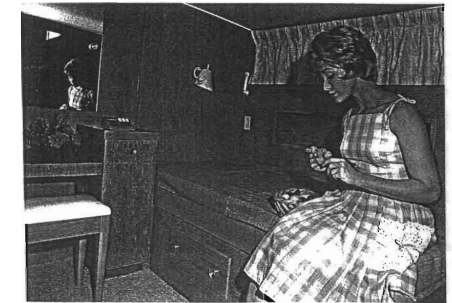
Master Stateroom Looking Aft
